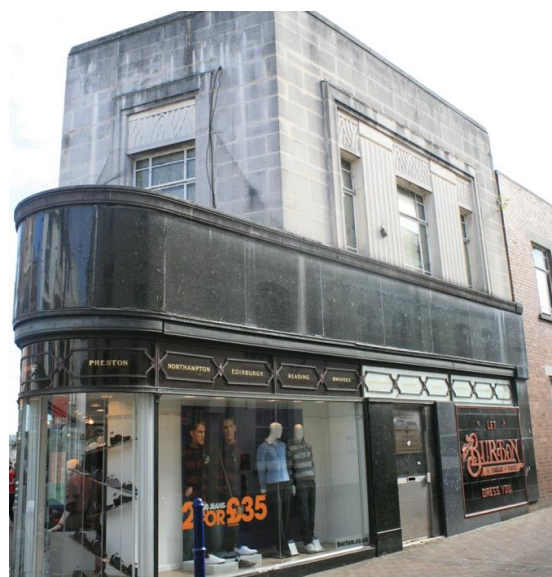
Fig.17 The Grade II listed Burton store shopfront – high quality materials, projected 'bow' plan and high quality lettering.
