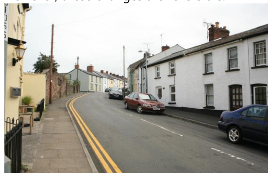
Fig.24 Victoria St – a common and consistent use of materials; painted render and natural slate roofs with red brick chimneys
