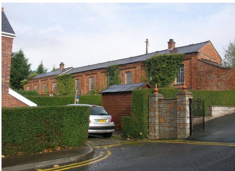
Fig.68 The Goods Building – a long brick range equivalent to two storeys in places (here seen from Hatherleigh Rd)
