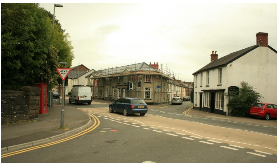
Fig.28 High quality townscape comprising listed and unlisted buildings define the junction of Brecon Rd & Commercial St
