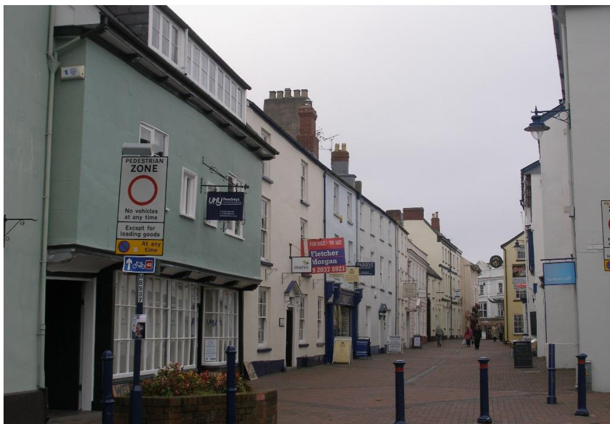
Fig.41 No 29 Nevill Street (in the foreground with the green frontage) – note the projecting upper floor indicating a timber frame behind the plastered façade
