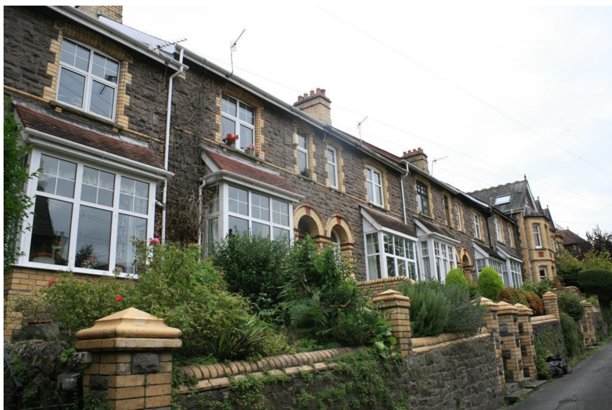
Fig.13 Stone boundary walls with buff brick copings are key features of this part of the conservation area
