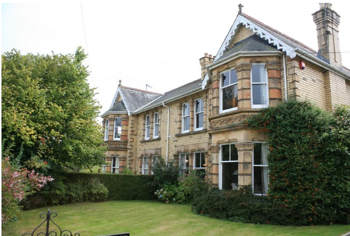
Fig.31 Yellow brick houses with decorative terracotta dressings and timber bargeboards.
