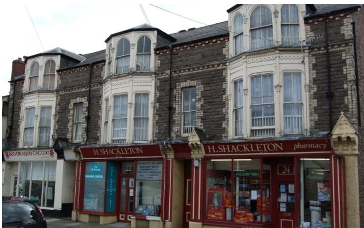
Fig.29 A rich palette of traditional materials is seen to this part of the conservation area (shops with accommodation above, Brecon Rd)
