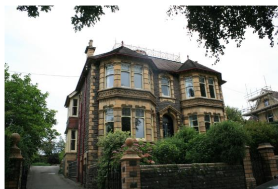
Fig.12 An eclectic mix of building materials to the villas in this part of the conservation area
