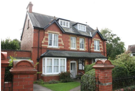
Fig.30 Avenue Rd characterised by large detached and semi-detached villas set in large plots with brick boundary walls and railings to the street frontage
