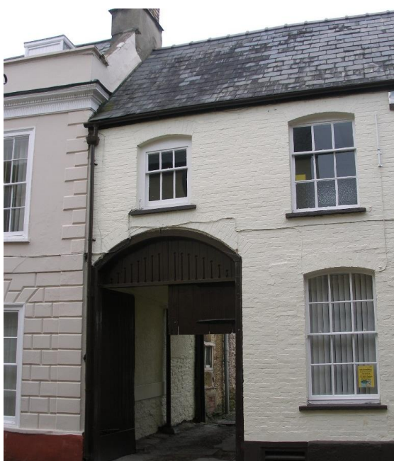
Fig.43 The end of the building in stucco plaster (with projecting quoins) is projecting forward of the adjacent painted brick building (with carriageway arch). This is a possible indication of refronting of an earlier stone building. The Older stone flanks of this building can be seen through the archway.
